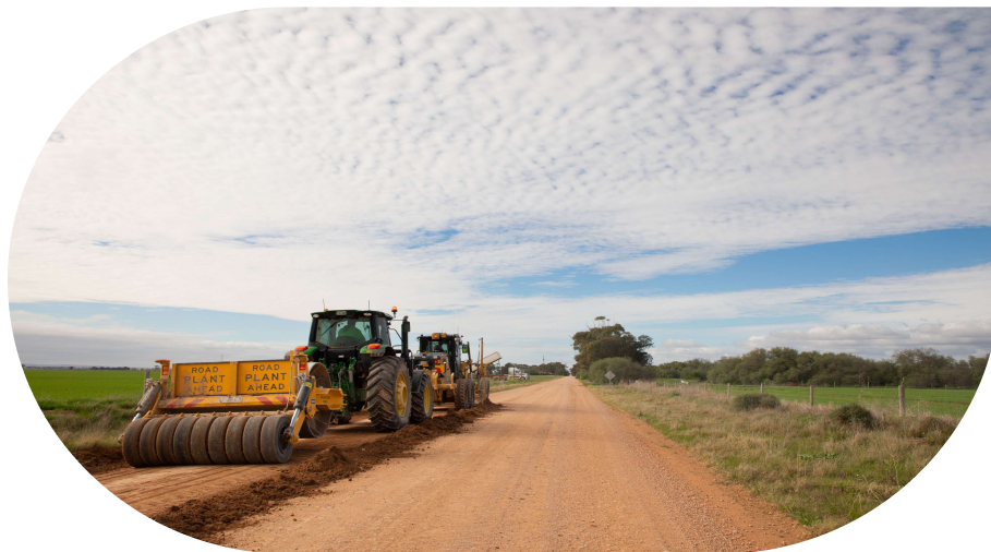
A typical Council rural unsealed road asset being resheeted.
