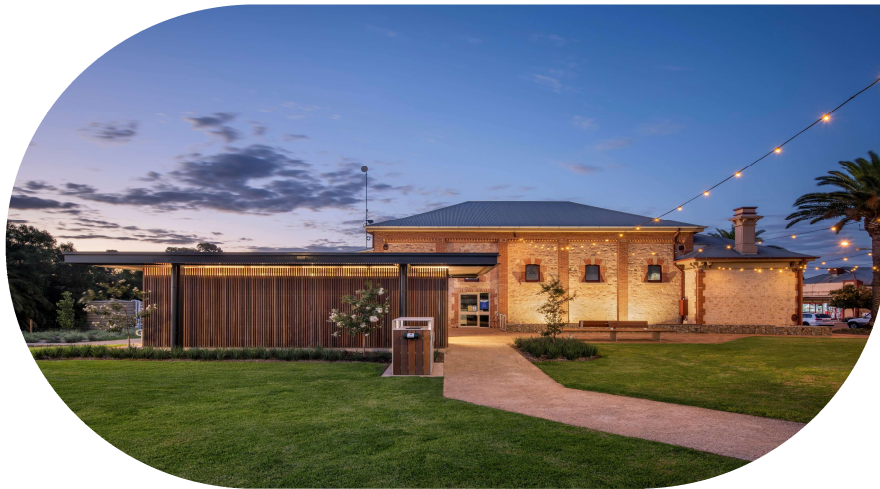
A typical Council building asset.
