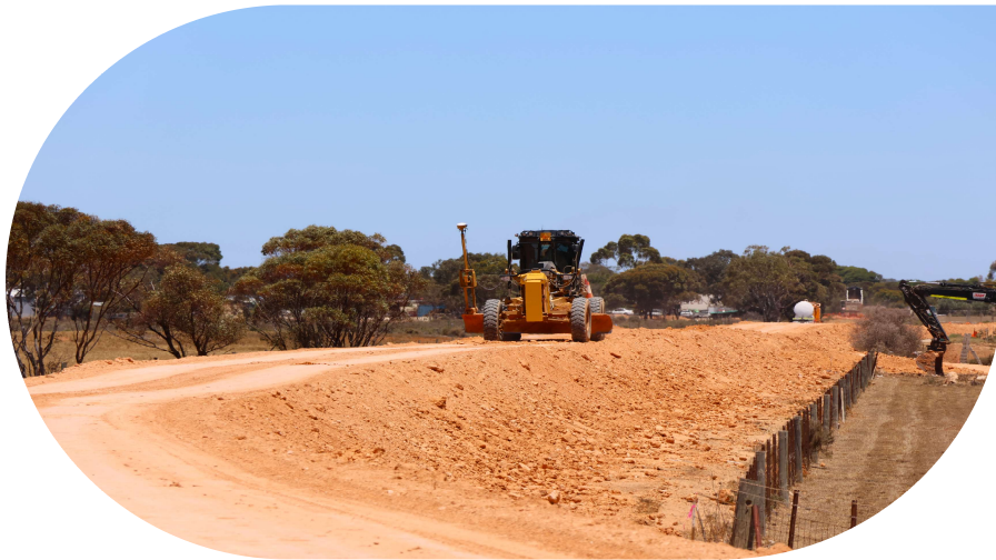
The Two Wells levee under construction.
